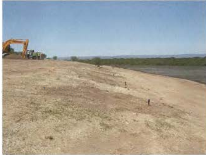
Pin Wells installed at the perimeter of the site to manage LFG emissions
