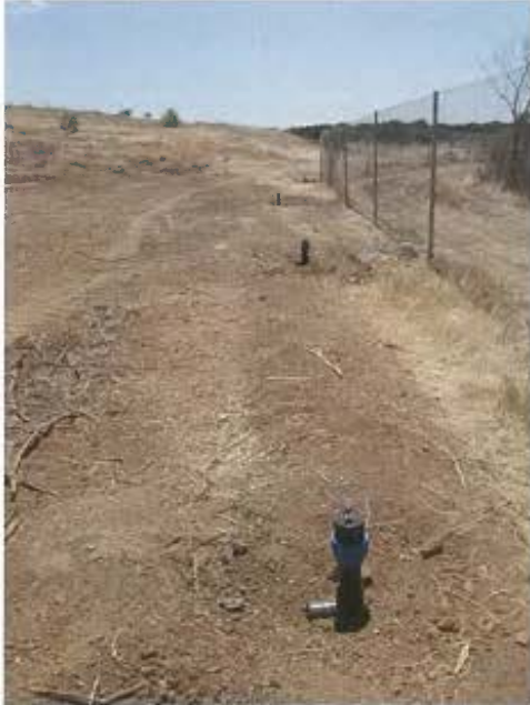
Pin Wells installed at the perimeter of the site to manage LFG emissions
